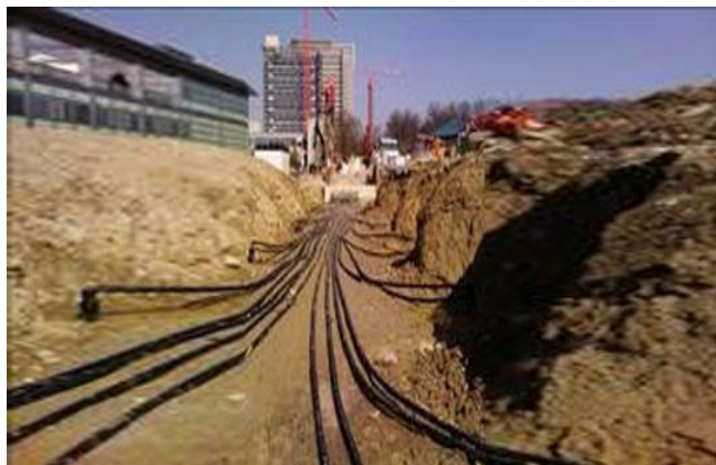
Fig 2: Science City Stores Warm Air from summer to Heat Buildings in Winter
