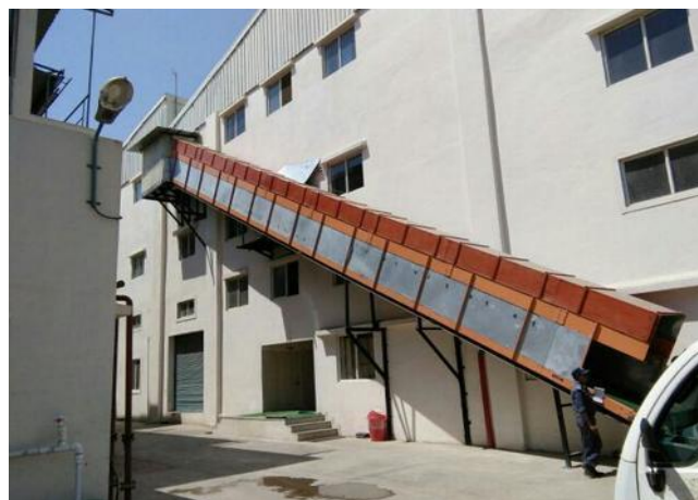
Fig 1: Gravitational Chute used for transportation in an Apparel Factory
