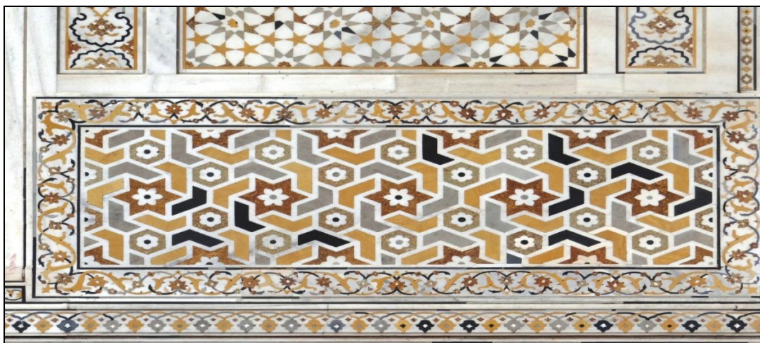
Fig 4: Etimad-ud-Daulah tomb in Agra, 1628 CE, celebration of 6 and 10 point geometrical patterns by inlay and carved marble through the facade of tomb
